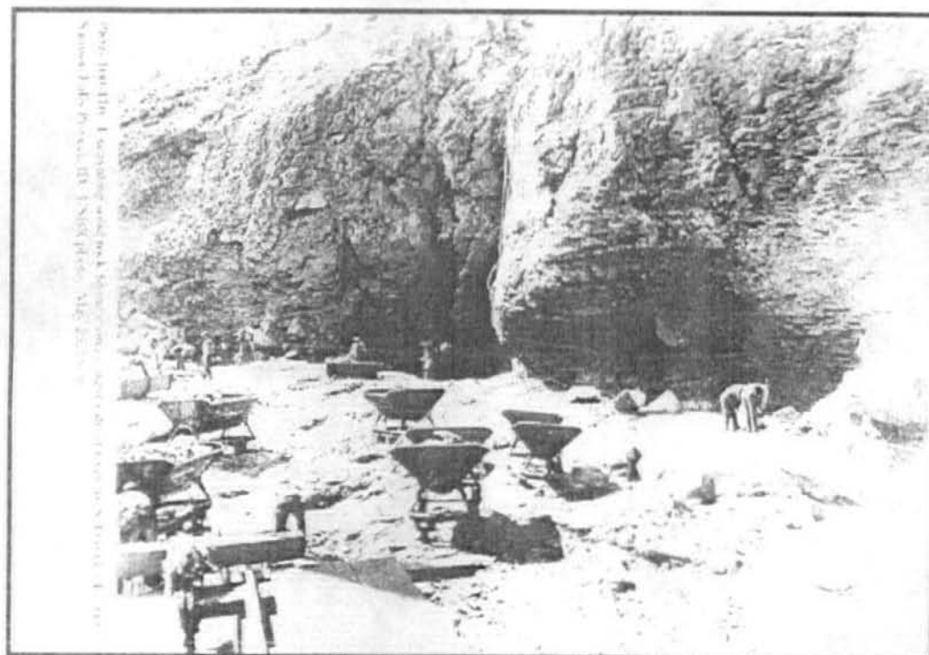
Excavation reaching bedrock May 25, 1909 (US Bureau of Reclamation Photograph).
