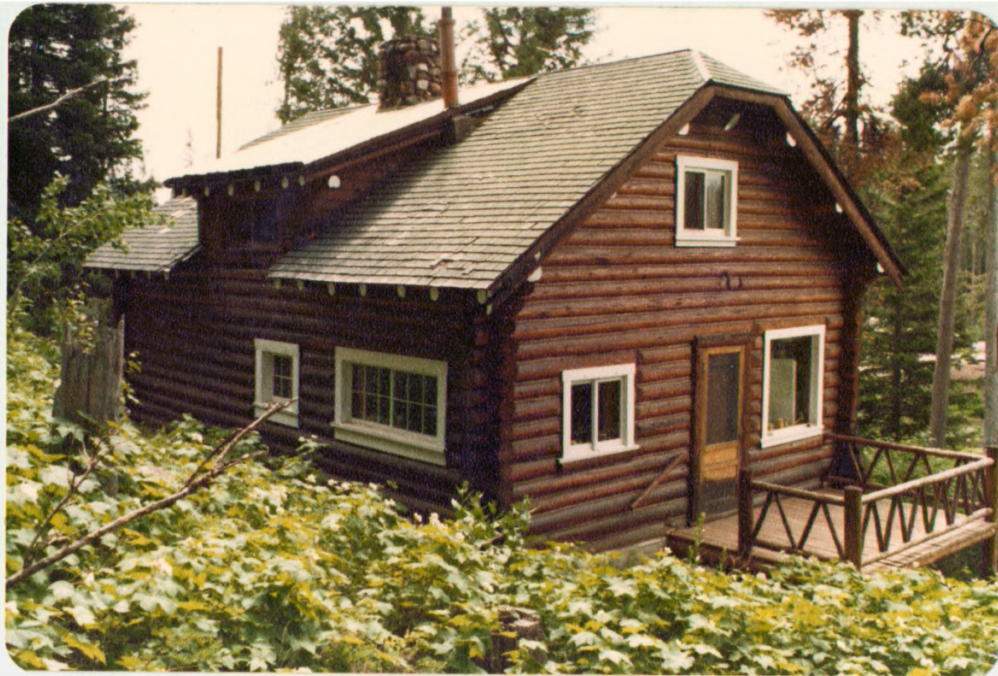
Fig. 6. Sack Cabin, northeast corner.
