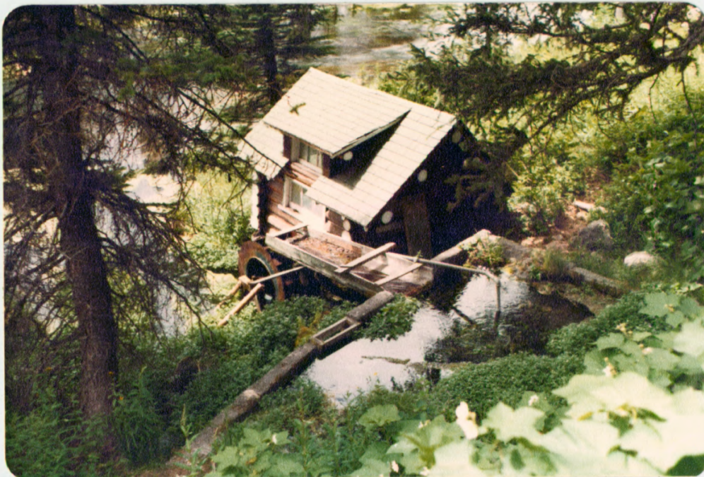
Fig. 7. Water-powered pumphouse (not in use).
