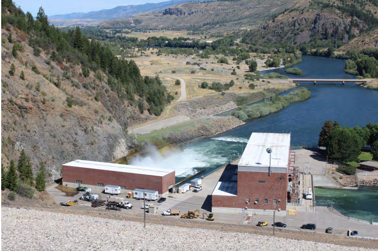
Photo 11 of 30. General view of gate house and powerplant. View to north.
