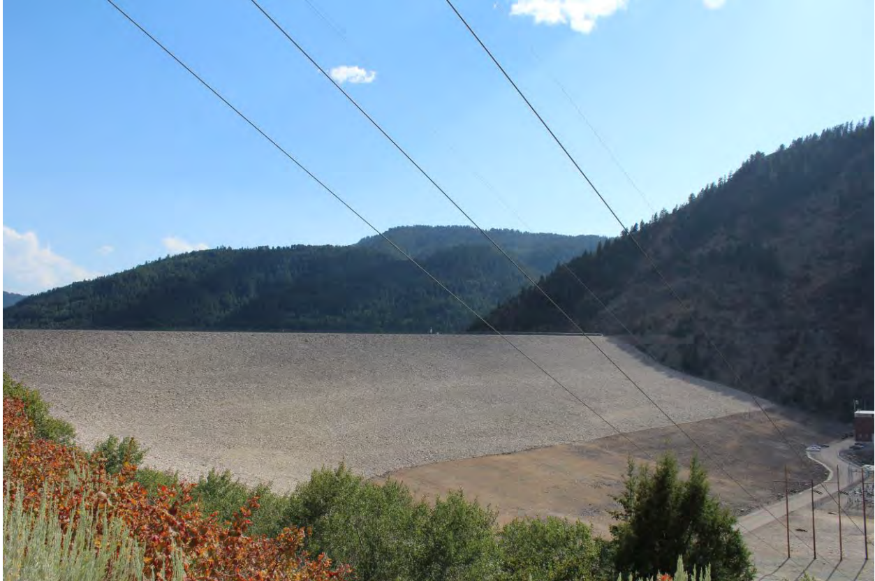
Photo 5 of 30. Dam, downstream slope. View to southwest.
