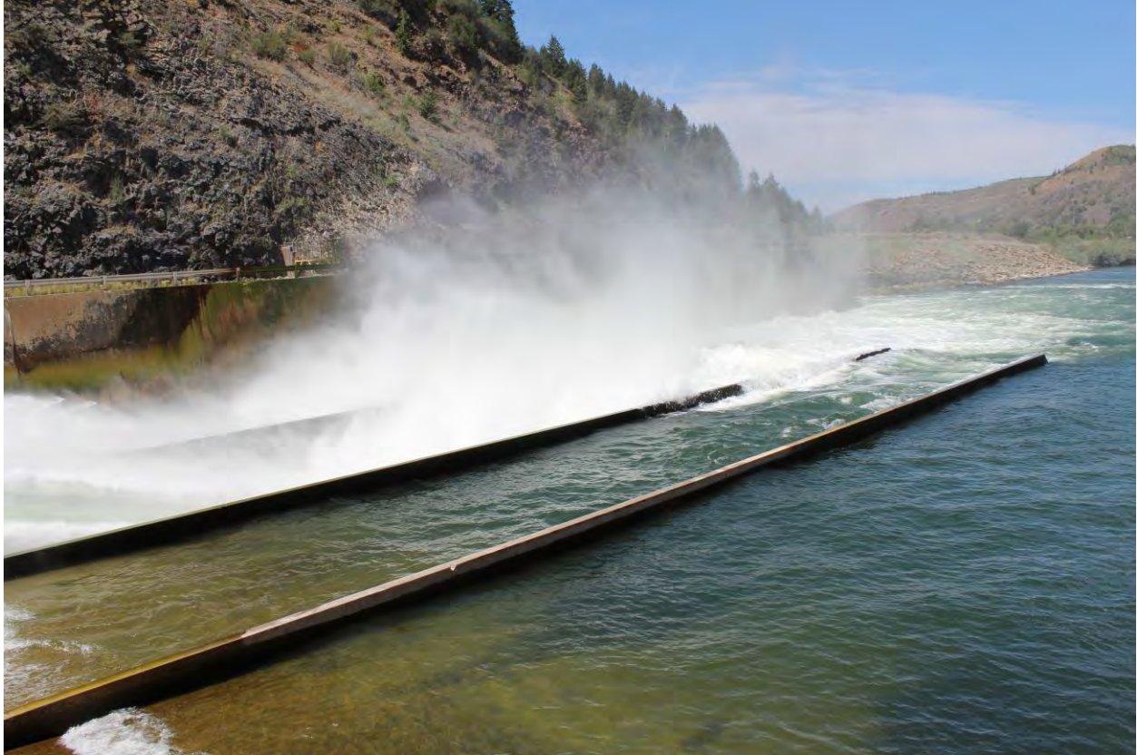
Photo 15 of 30. Stilling basin dividing walls. View to northwest.
