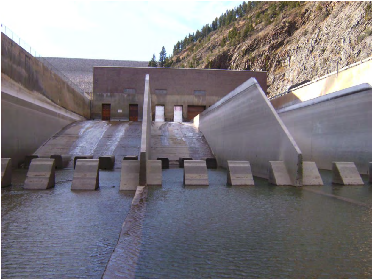
Figure 13. Stilling basin with upper chute, dividing walls and chute blocks visible.
