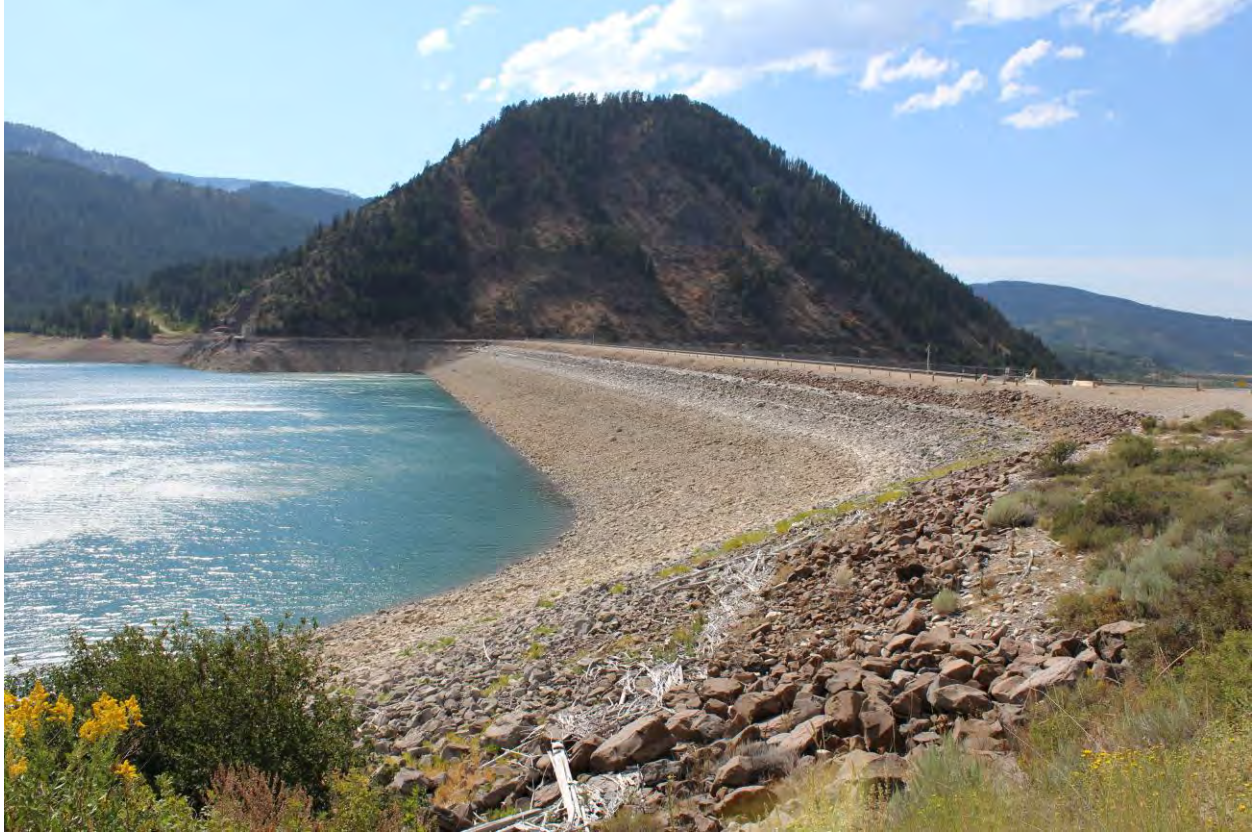
Photo 6 of 30. Dam, upstream slope. Calamity Point in background. View to west.
