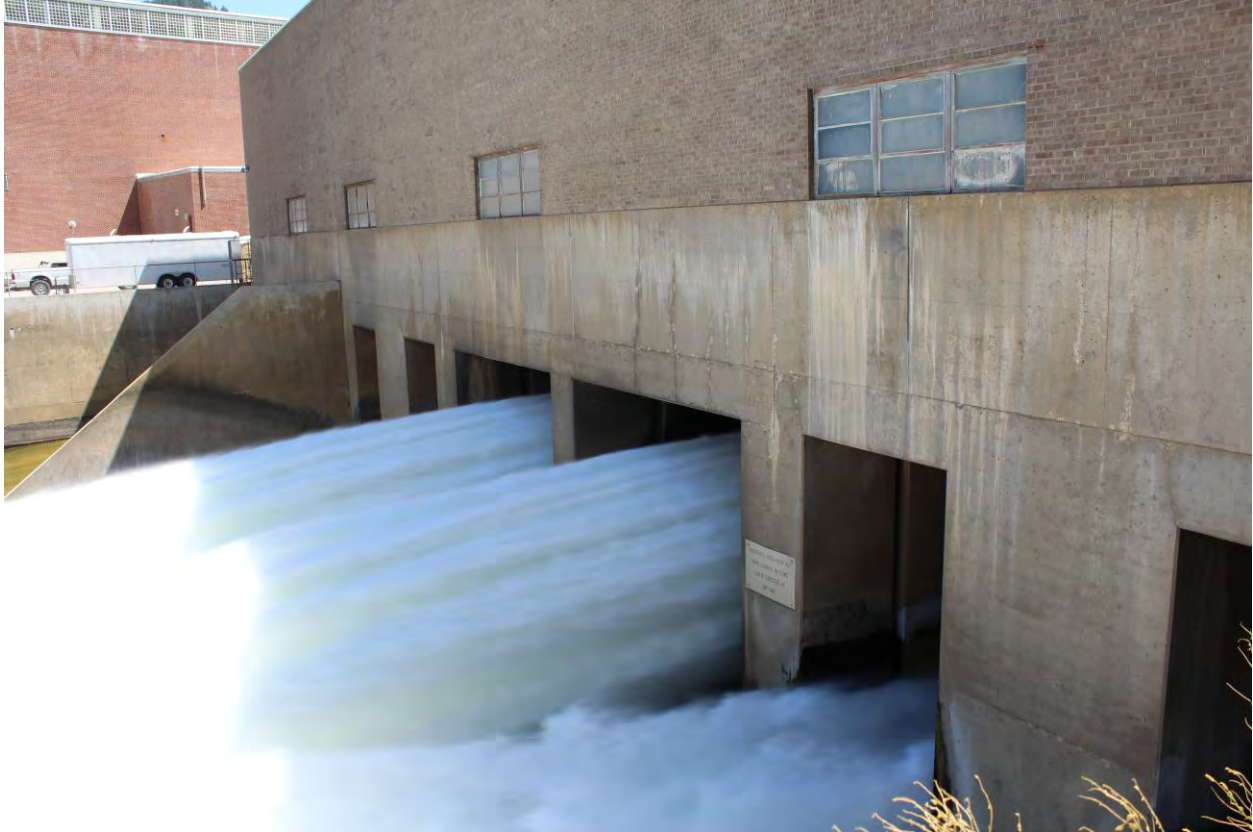
Photo 13 of 30. Gate house discharge area. View to southeast.
