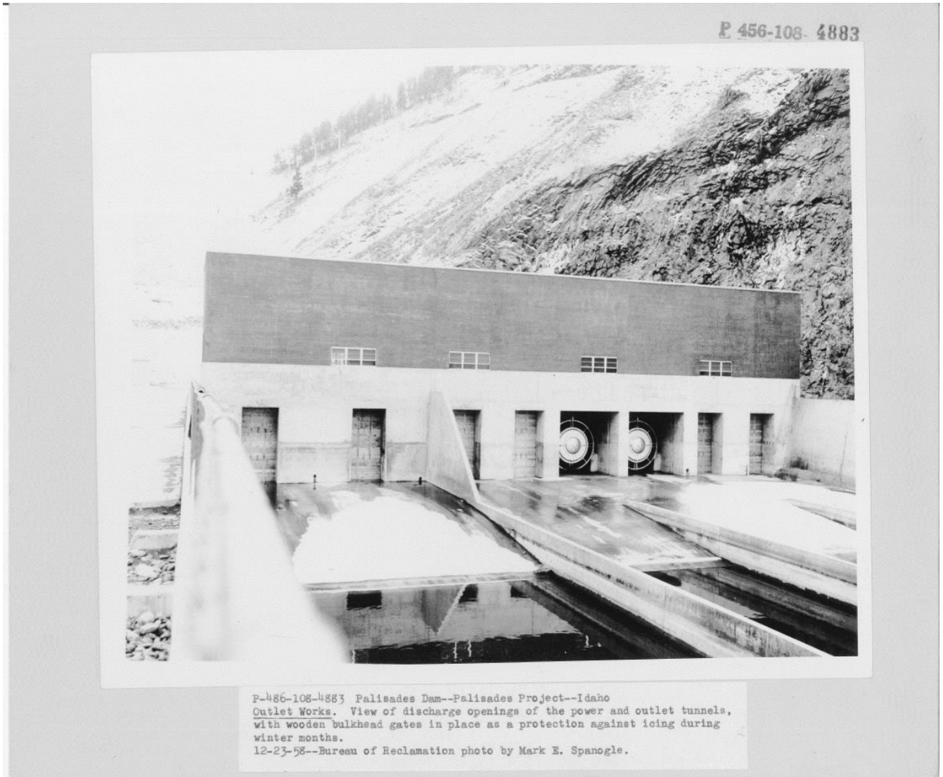
Figure 12. Gate house, discharge openings of the power and outlet tunnels and stilling basin in foreground, 1958.
