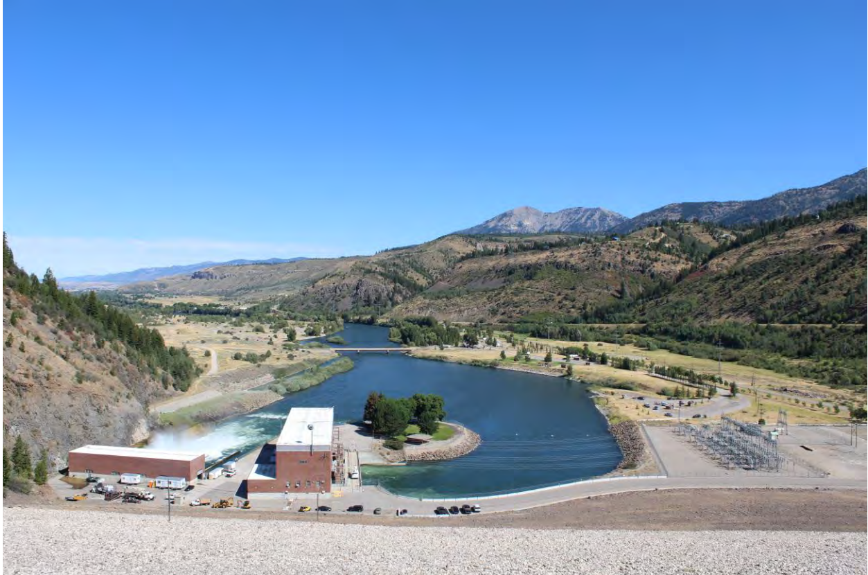
Photo 3 of 30. General view of gate house, powerplant, Vista Park, tailrace and switchyard. View to north.
