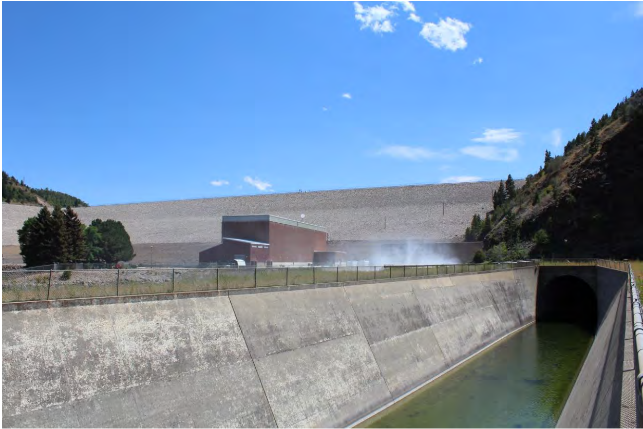
Photo 27 of 30. Spillway channel. View to south.
