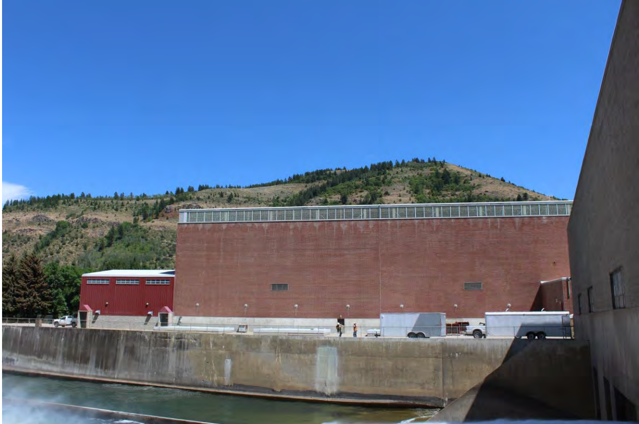
Photo 19 of 30. Powerplant west elevation with stilling basin in foreground. View to east.
