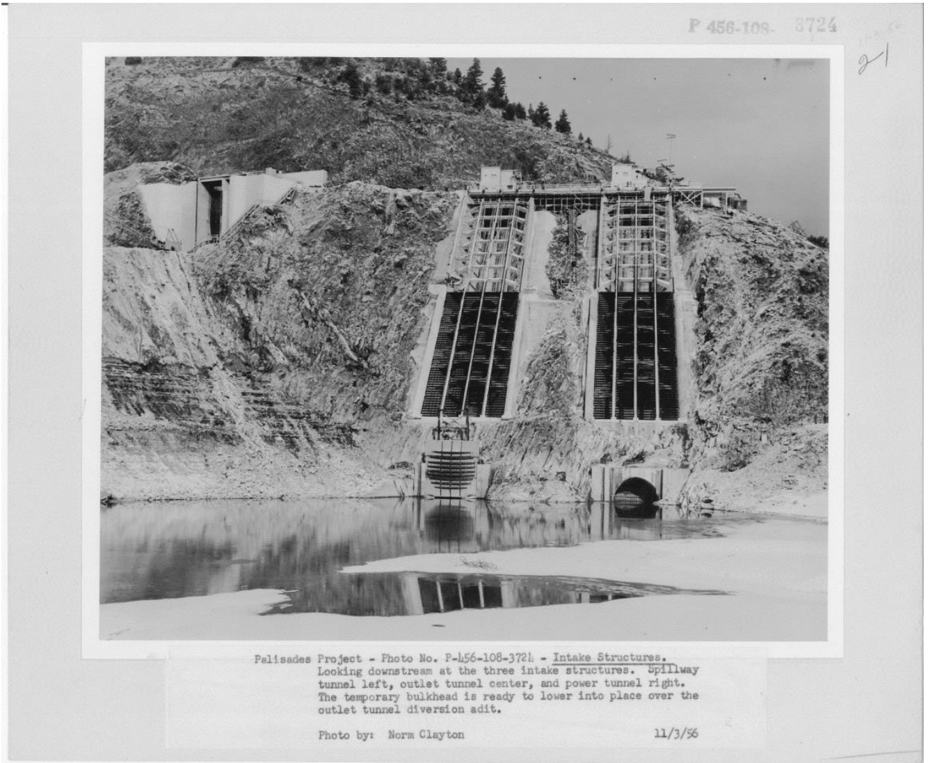
Figure 8. Intake Structures, looking downstream. The spillway is on the far left, the outlet tunnel in the center and the power tunnel on the right. 1956
