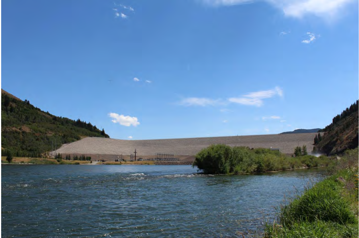
Photo 1 of 30. General view of dam and tailrace. View to south.
