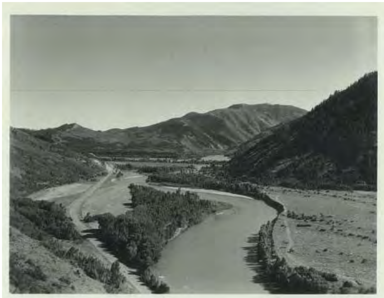
Figure 5. Dam site prior to construction looking upstream, July 1949.
