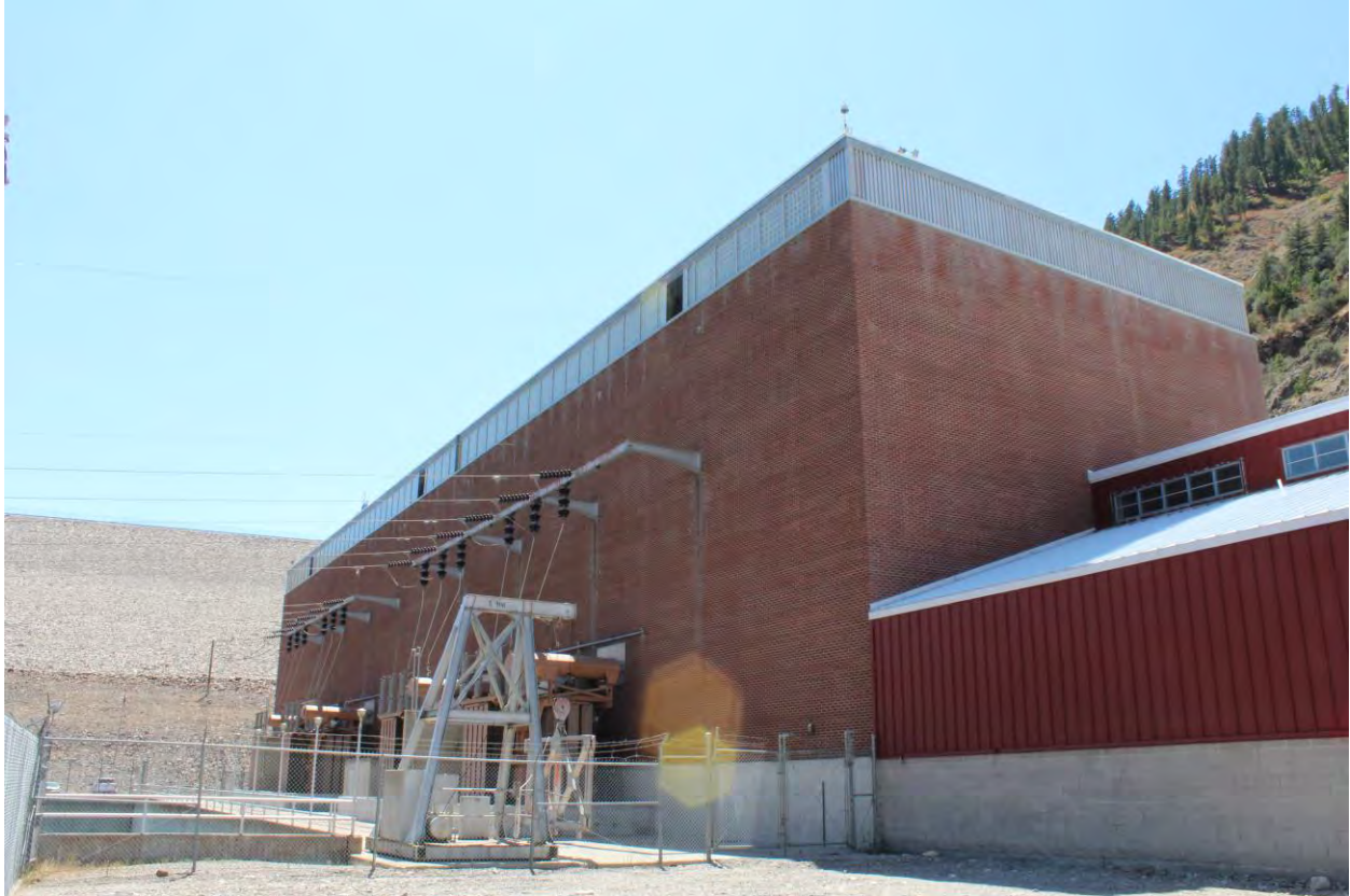
Photo 17 of 30. Powerplant transformer deck. View to southwest.
