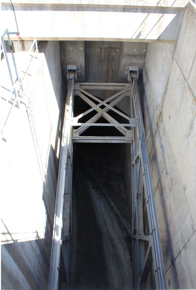
Photo 26 of 30. Spillway, radial arms of the spillway gate. View to north.
