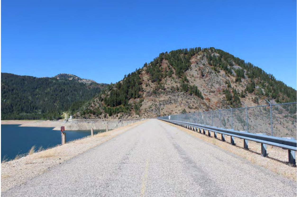
Photo 7 of 30. Dam, crest road on top of dam. View to west.
