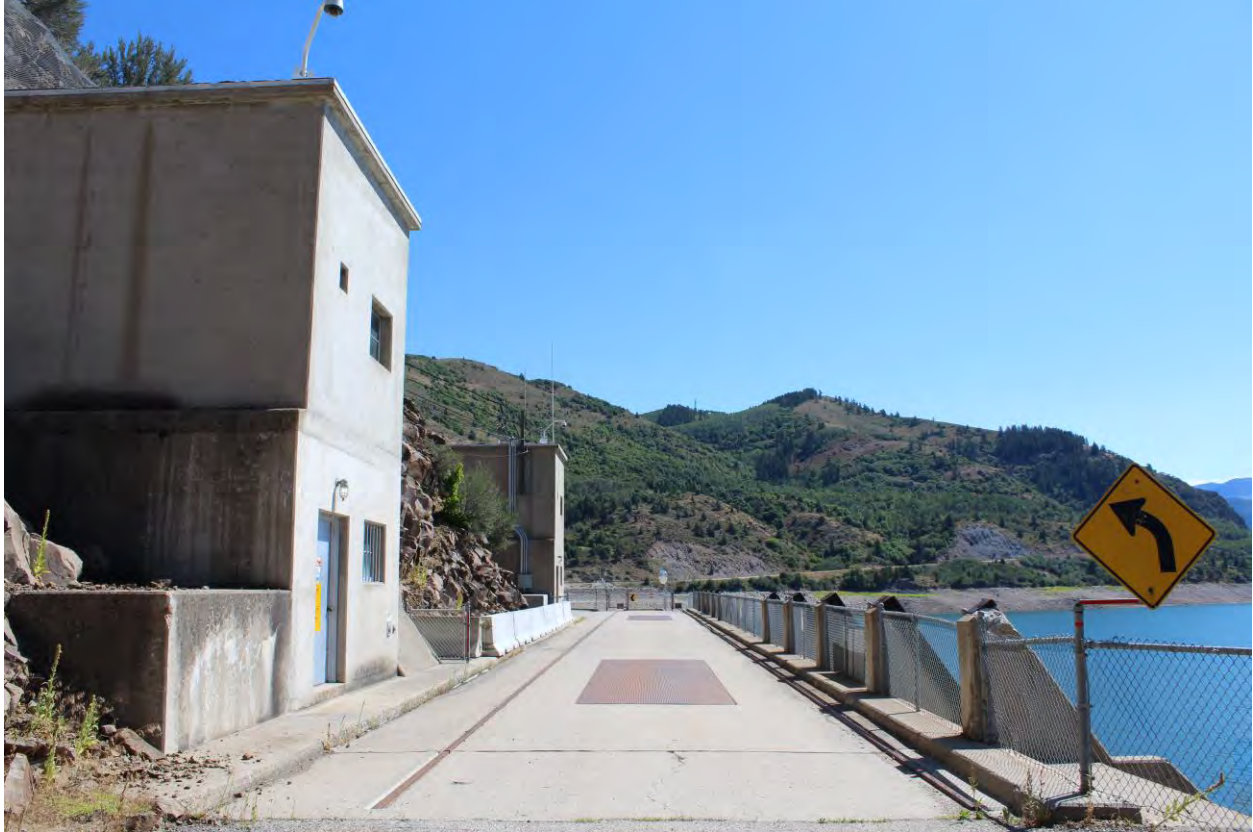
Photo 9 of 30. Bridge crossing intake structures; intake gate structures on left. View to east.
