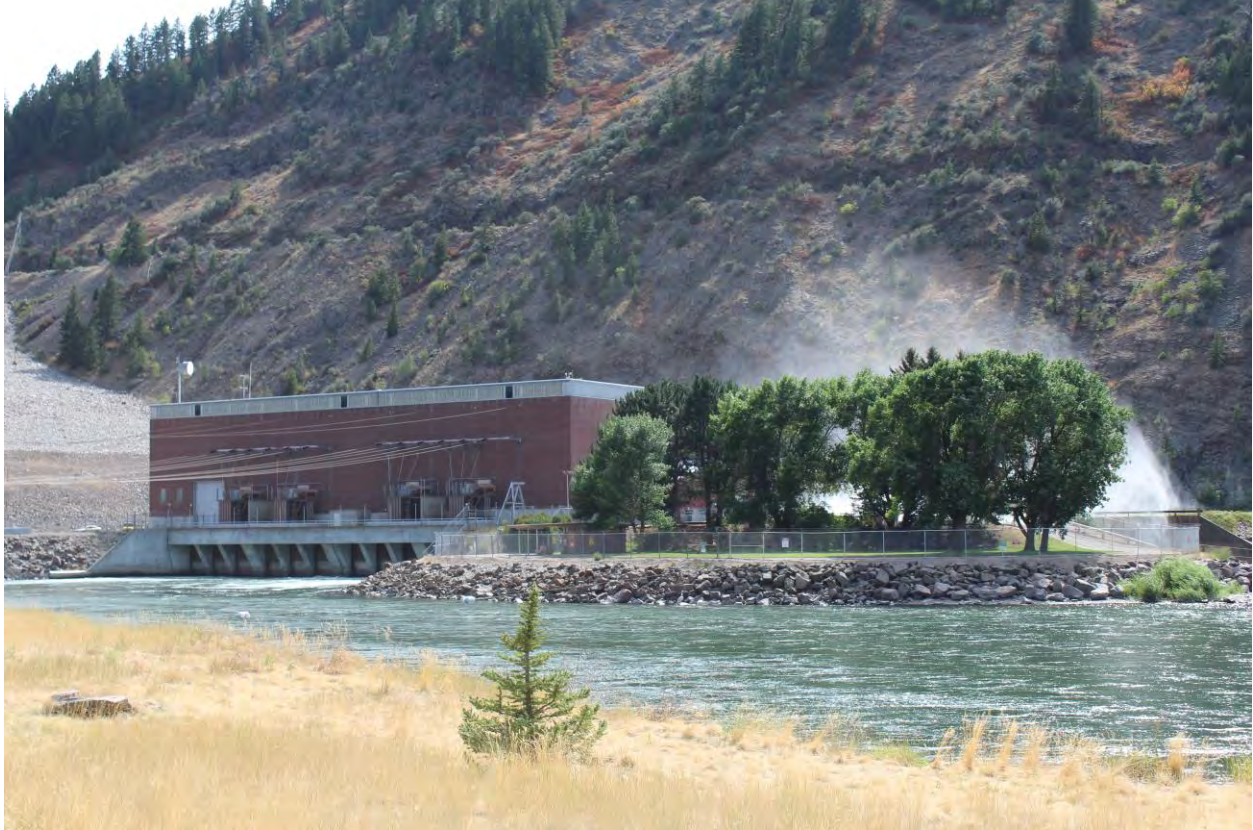
Photo 16 of 30. Powerplant transformer deck and Vista Park. View to southwest.
