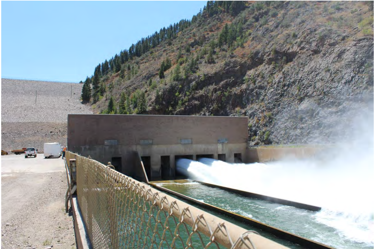
Photo 12 of 29. Gate house discharge area and dividing walls of stilling basin. View to southwest.
