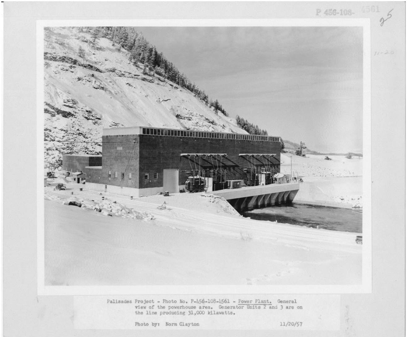
Figure 10. Powerplant, view of transformer deck, 1957.
