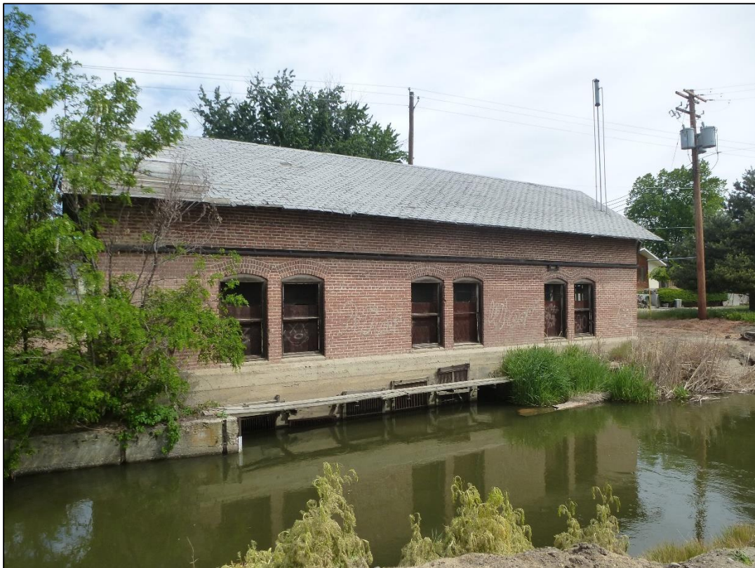
Photograph 12 of 25 South elevation, view looking NE
