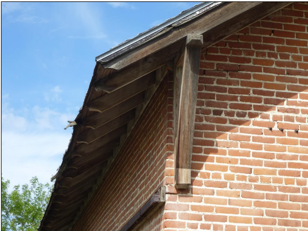
Photograph 8 of 25 Detail view, knee braces and exposed rafter tips, façade and south elevation
