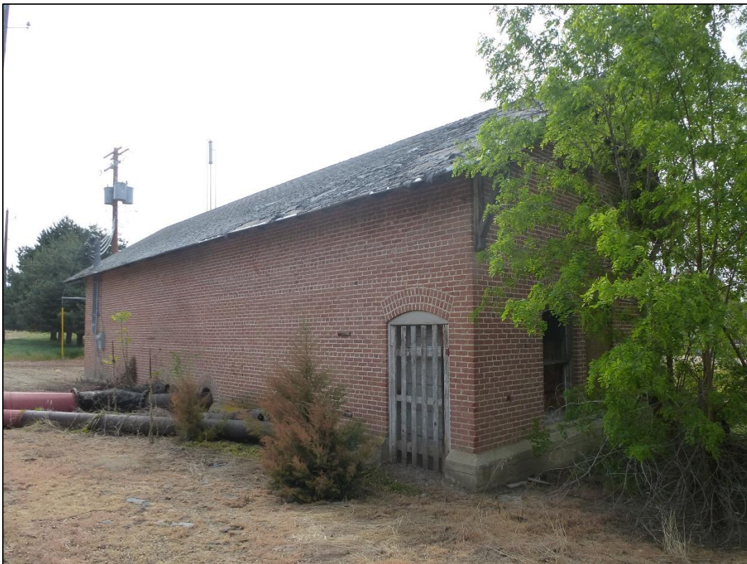
Photograph 4 of 25 North elevation and west elevation, view looking SE
