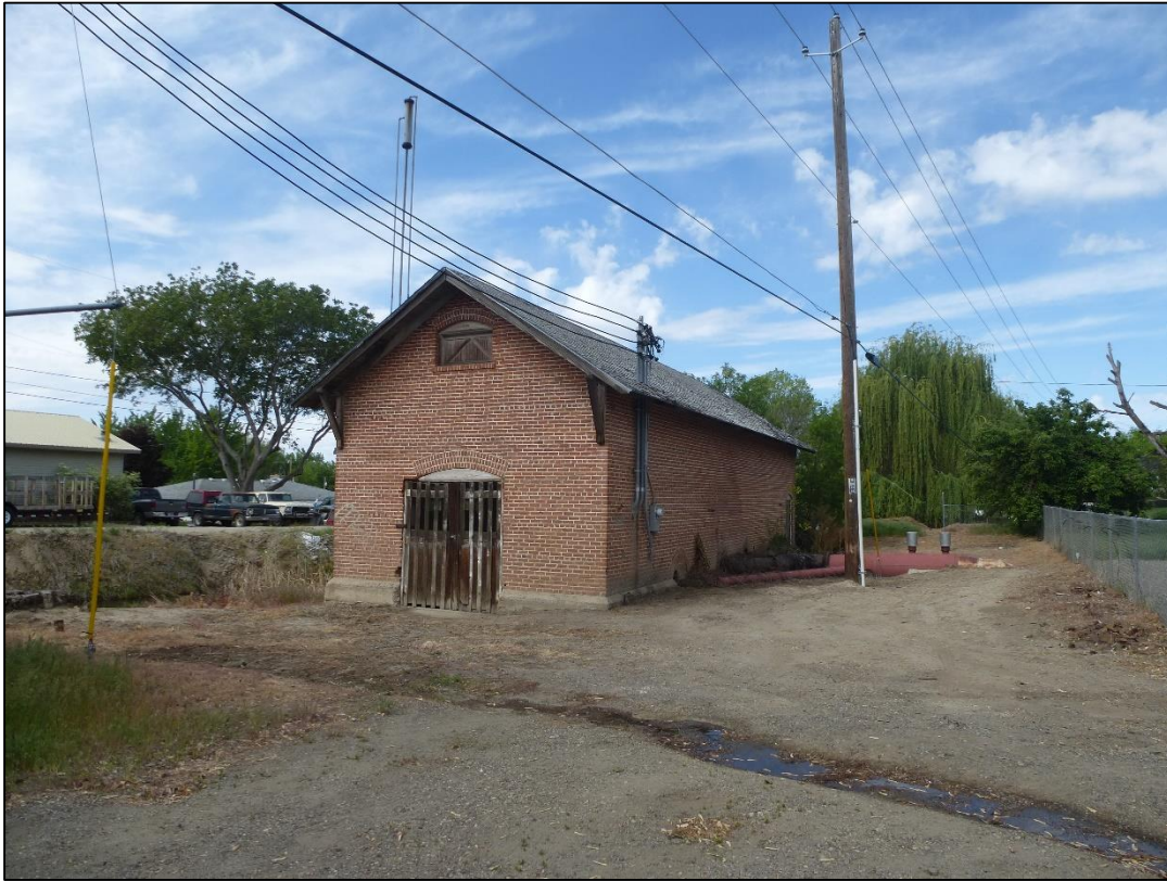
Photograph 3 of 25 Façade (east elevation) and north elevation, view looking SW
