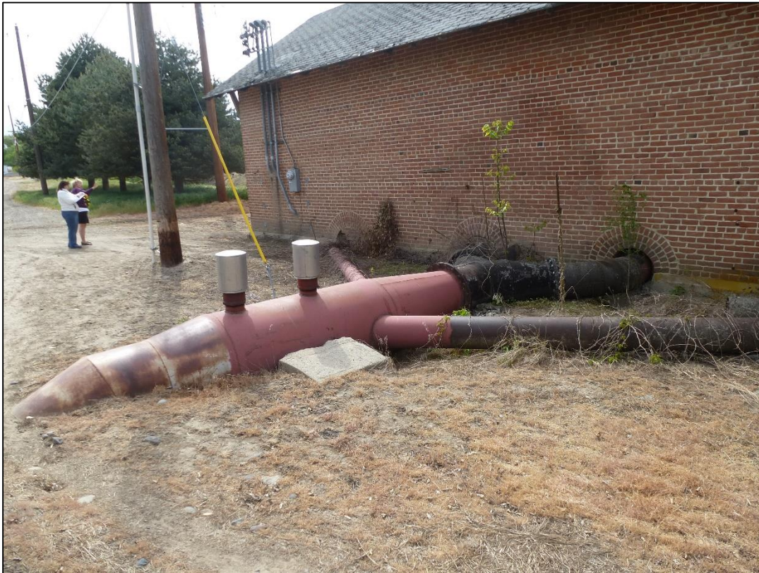
Photograph 10 of 25 North elevation, outlet pipes, view looking SE
