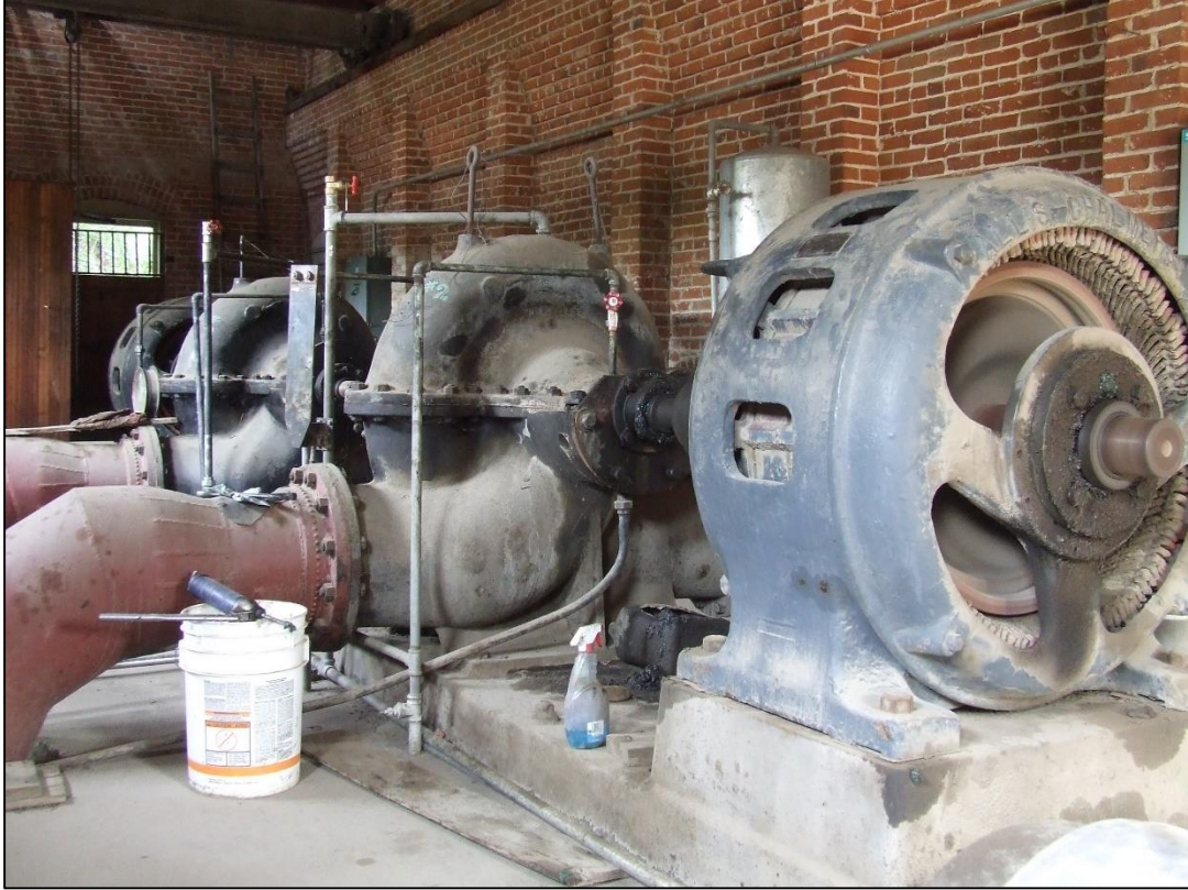
Photograph 15 of 25 Interior, view looking NW
