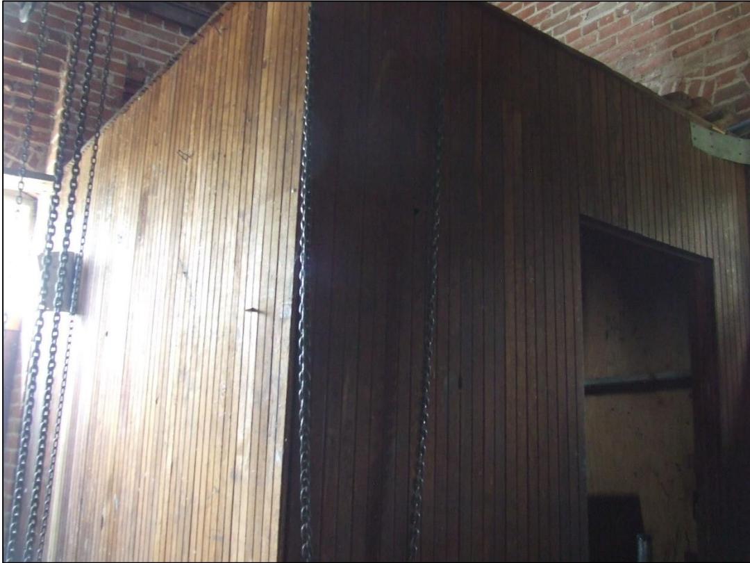
Photograph 21 of 25 Enclosed storage room, southwest corner of building
