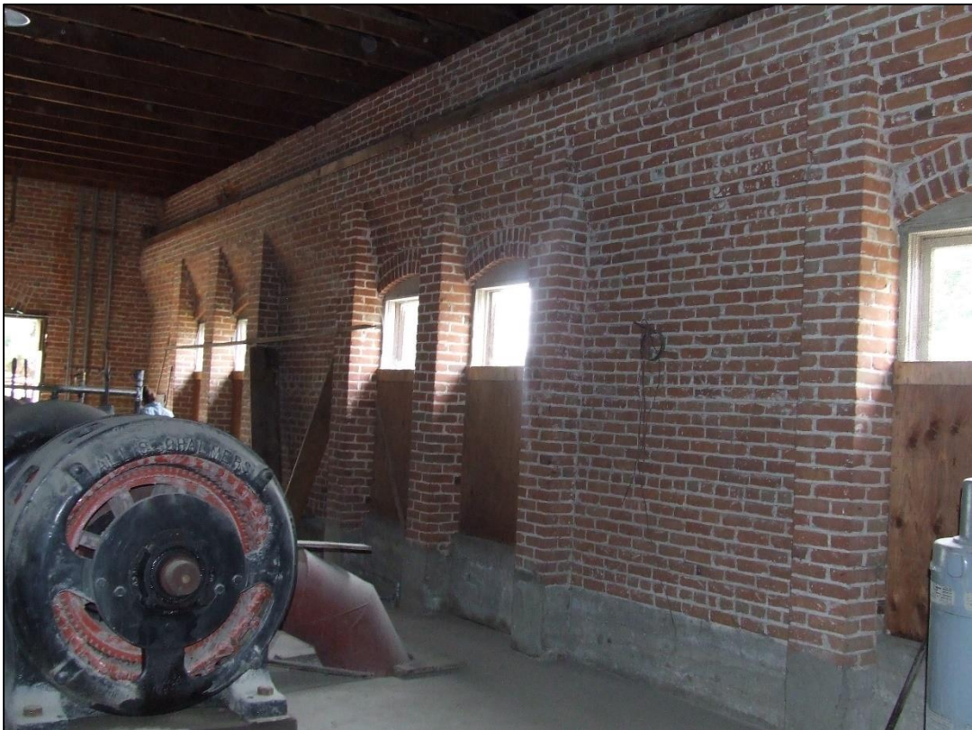
Photograph 20 of 25 South wall, view looking SE
