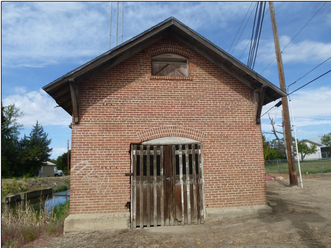
Photograph 2 of 25 Façade (east elevation), view looking W
