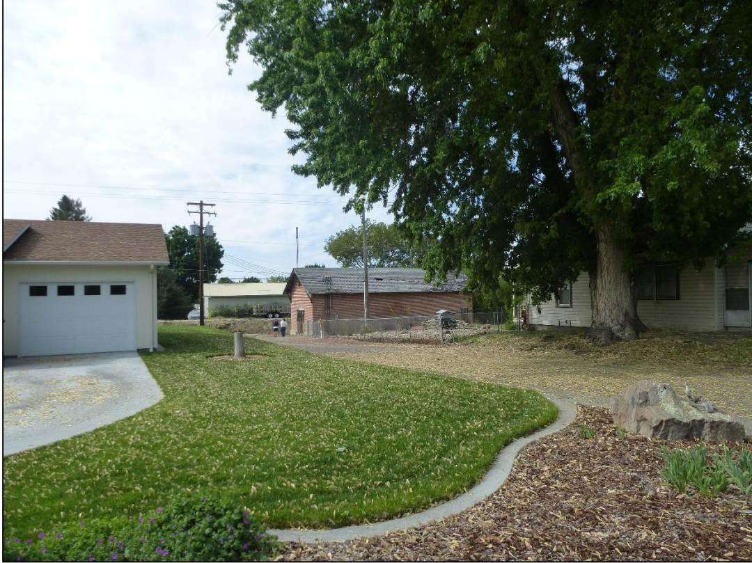
Photograph 25 of 25 Pump house from the intersection of Short Street and Fairview Avenue, view looking southwest.
