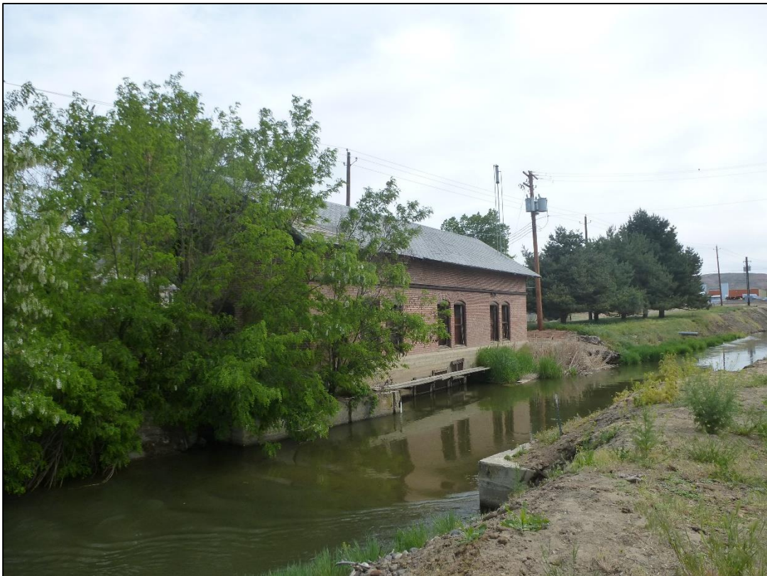
Photograph 6 of 25 South elevation, view looking NE
