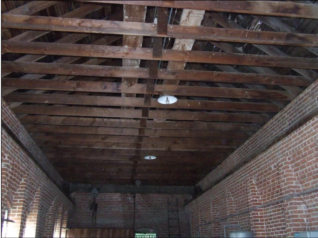
Photograph 17 of 25 Interior view of roof and upper walls, view looking W
