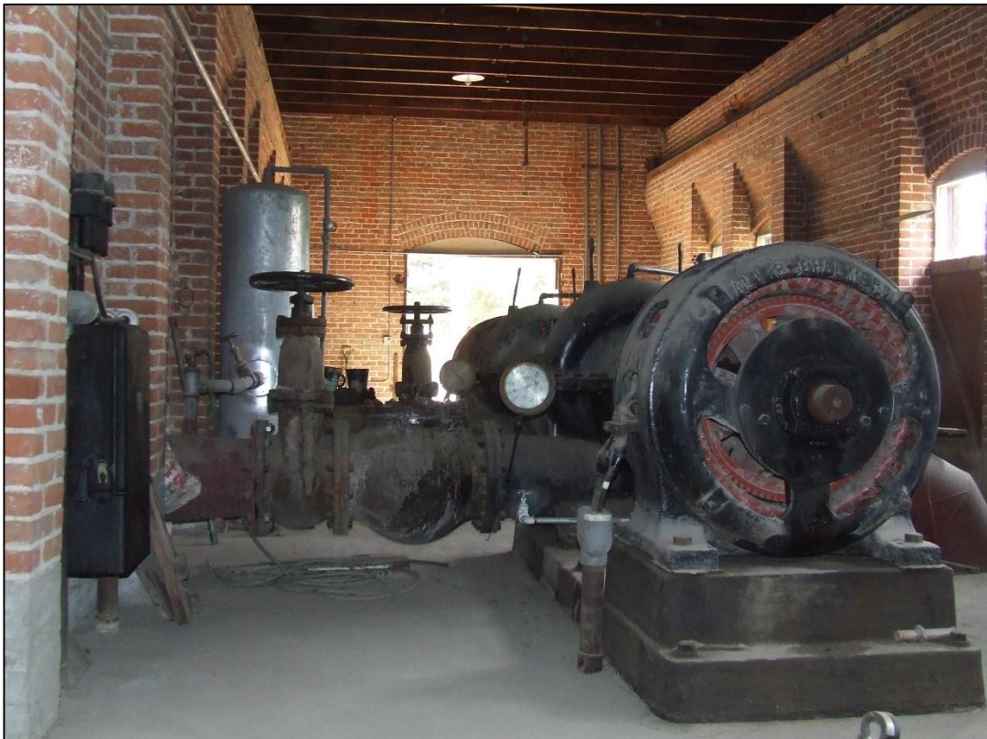
Photograph 14 of 25 Interior from rear of building, view looking E
