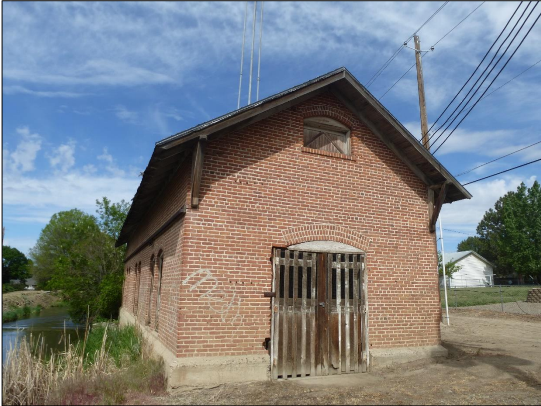
Photograph 1 of 25 Façade (east elevation) and south elevation, view looking W
