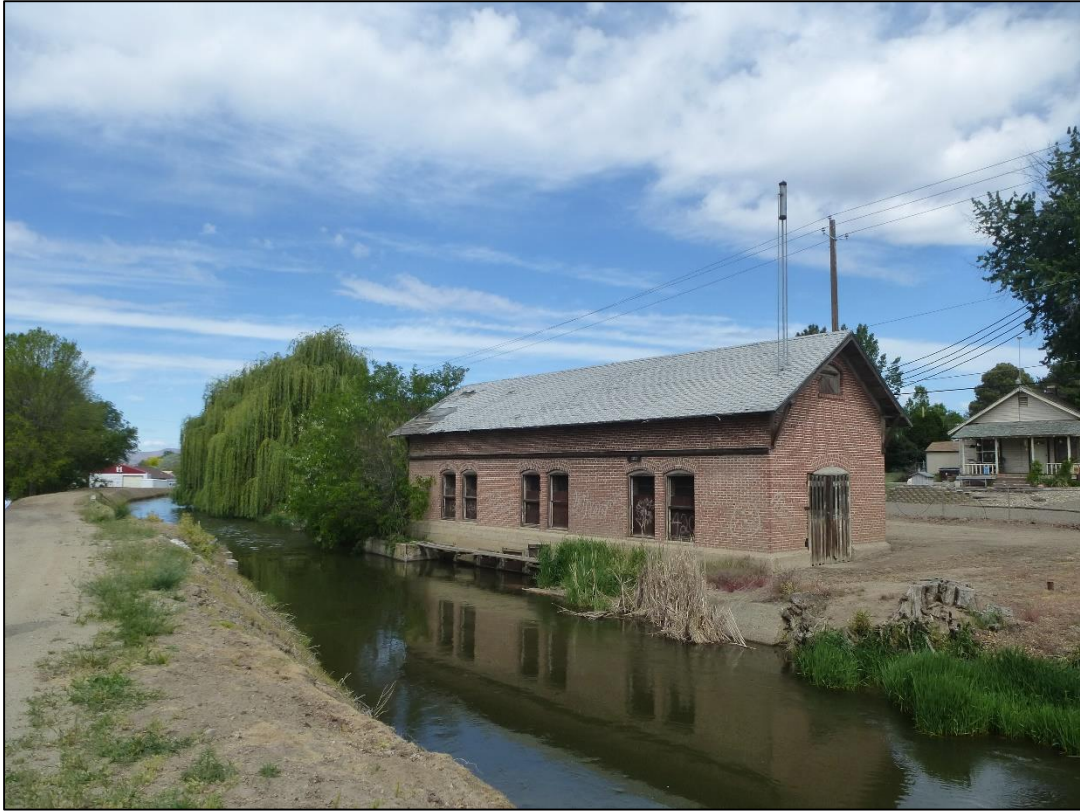
Photograph 5 of 25 Façade (east elevation) and south elevation, view looking NW
