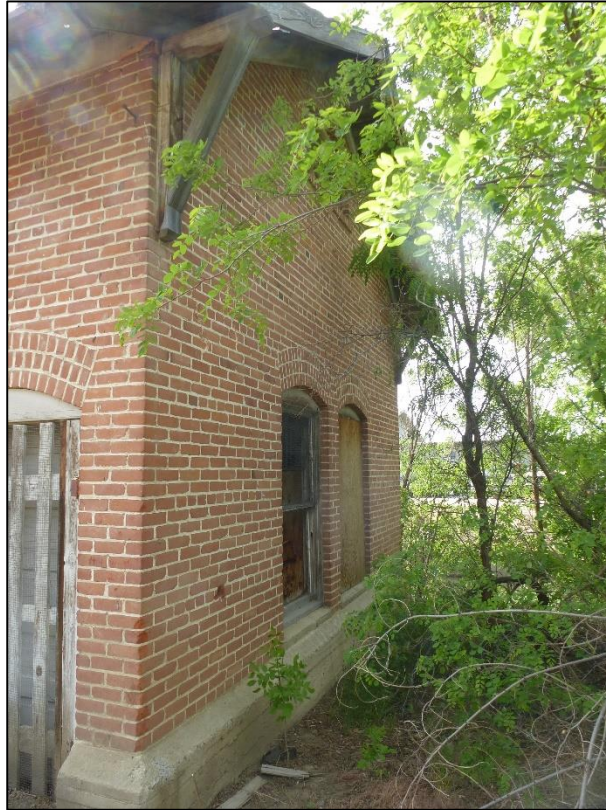
Photograph 11 of 25 West elevation, view looking S
