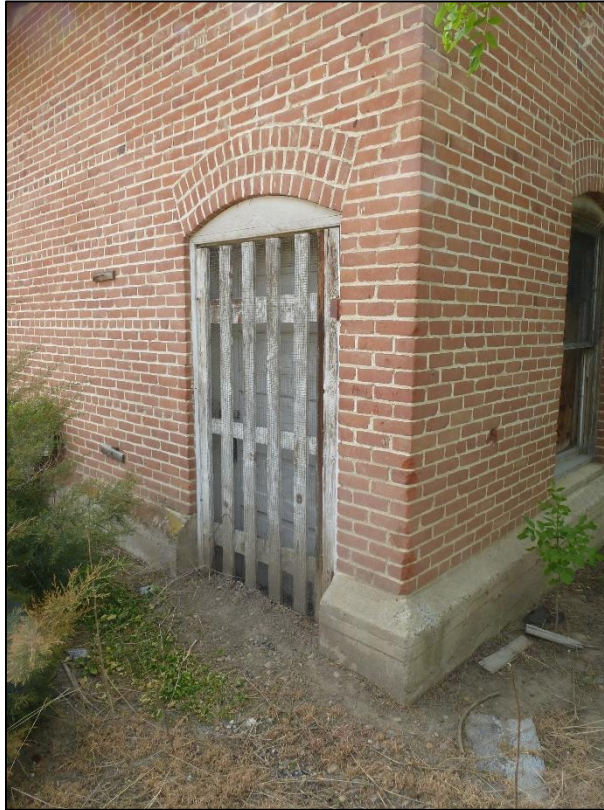
Photograph 9 of 25 Door, north elevation
