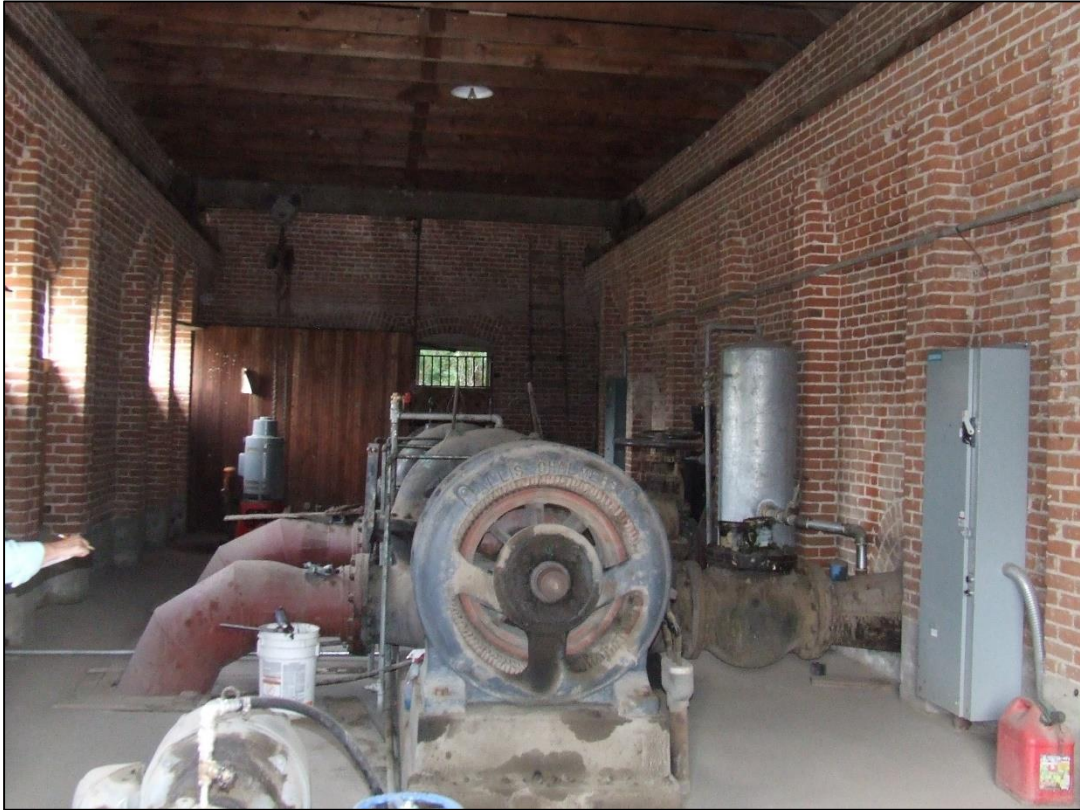
Photograph 13 of 25 Interior from main entrance, view looking W
