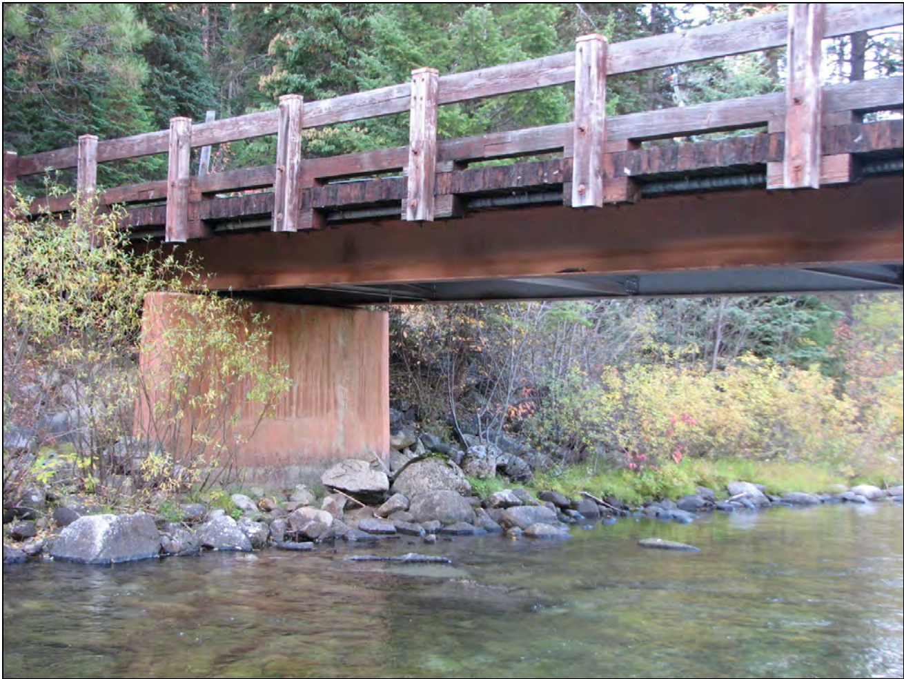
Photo 0008 Looking north-northwest to the I-beam bridge.
