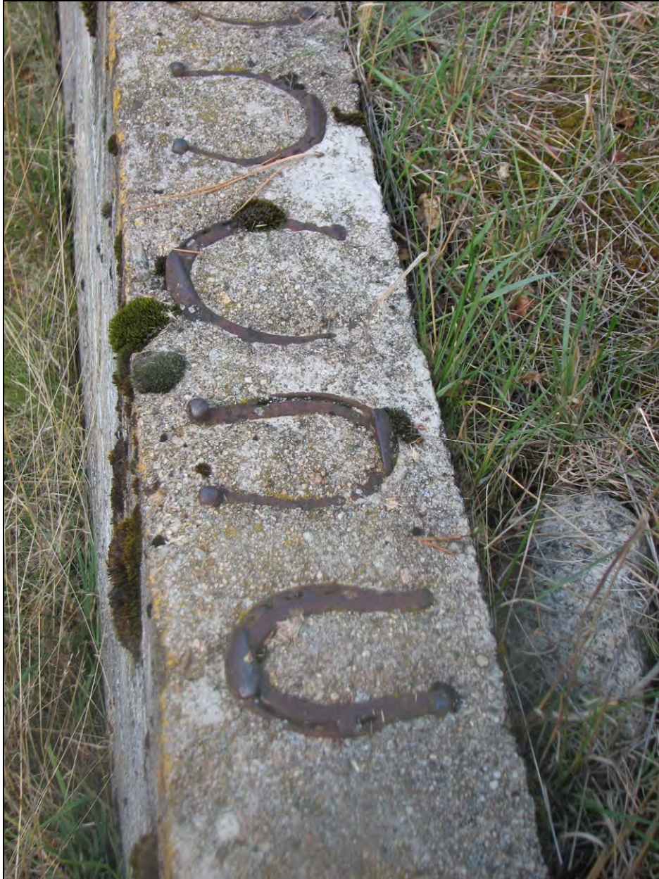
Photo 0027 Detail photo of the mule and horse shoos embedded in the stock loading ramp adjacent to the Barn.
