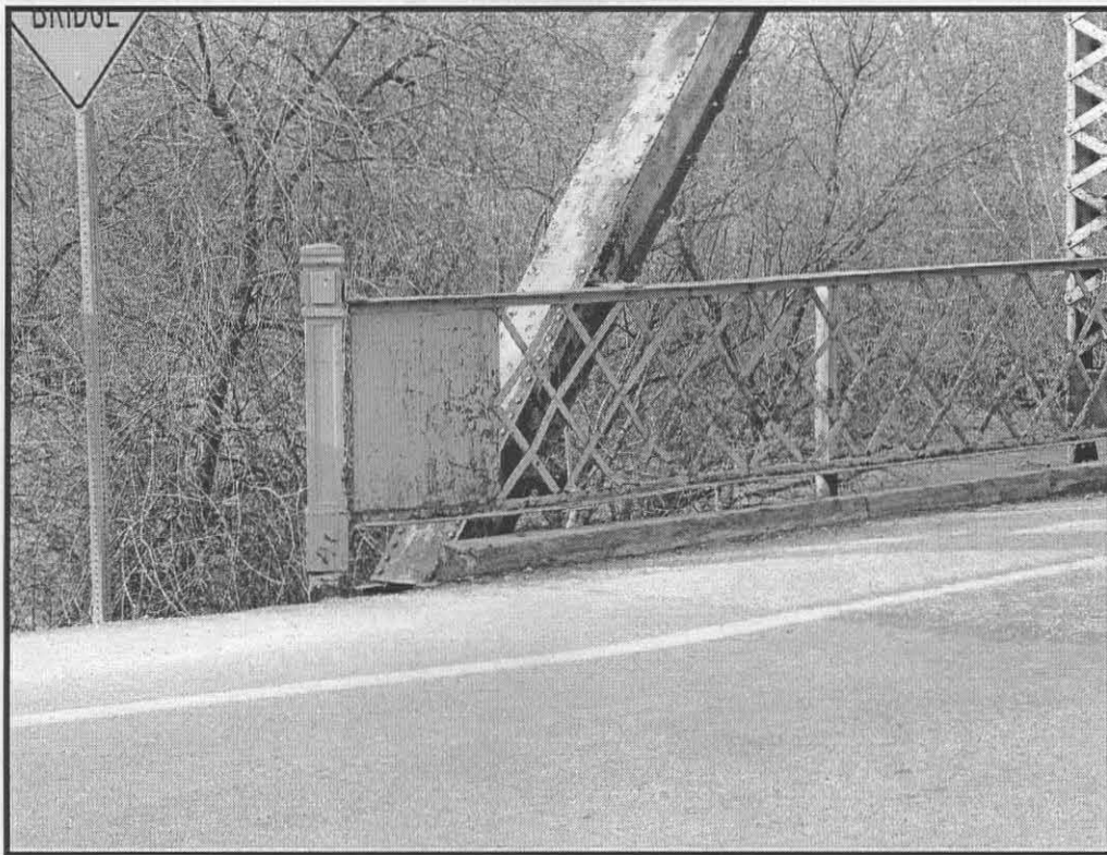
Original guard rail detail on east end of bridge.
