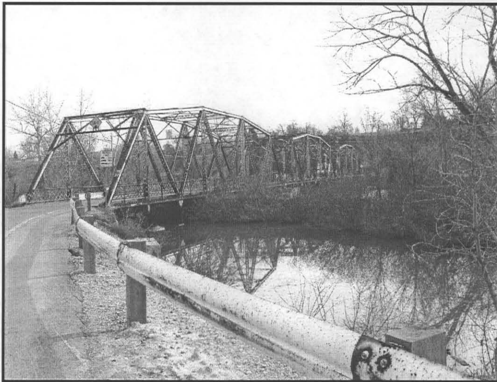
Boise River and Canal Bridge west side viewed to the northeast.
