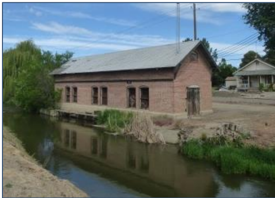
Institute Canal Company Pump House, Weiser
