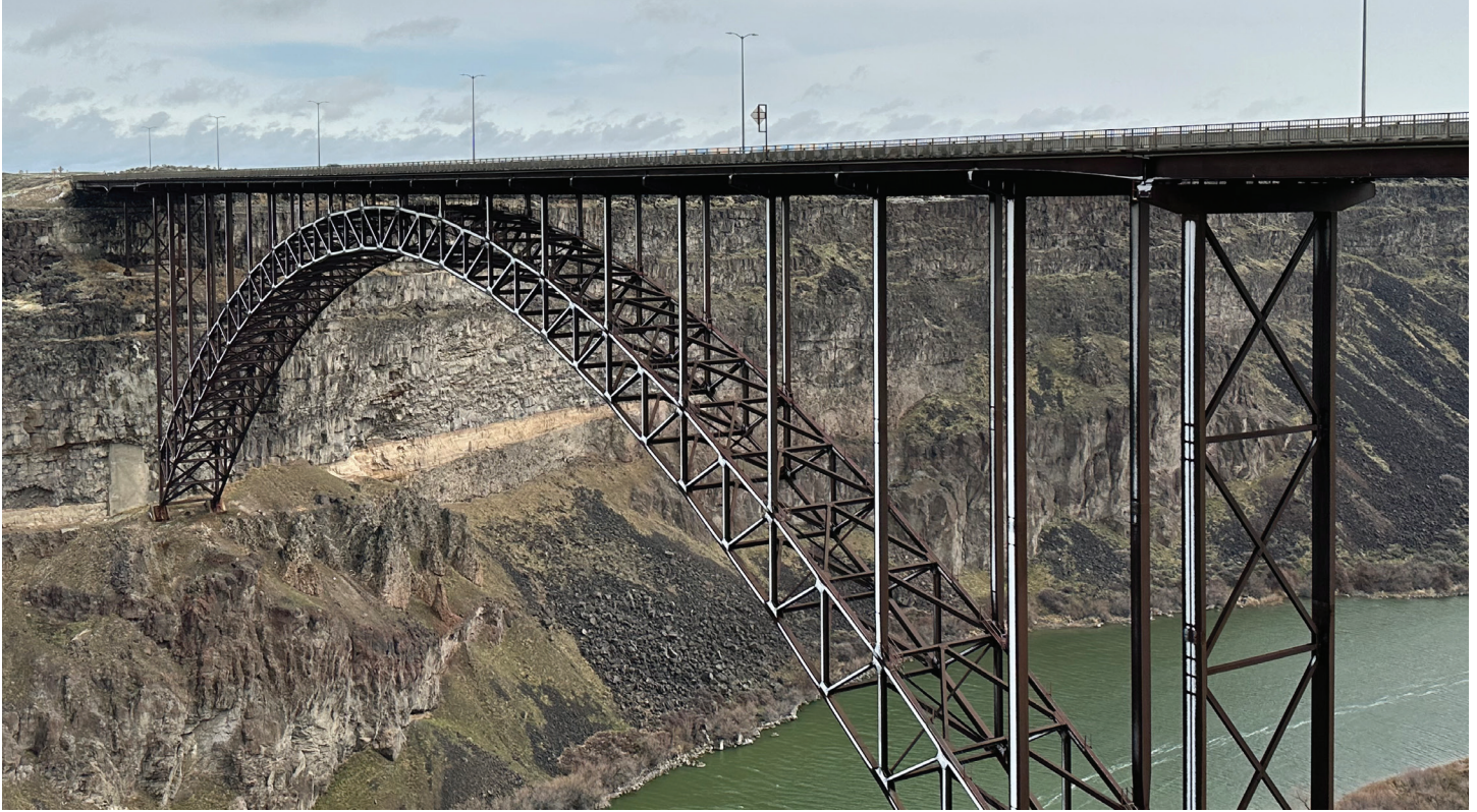
Perrine Memorial Bridge Twin Falls, ID
