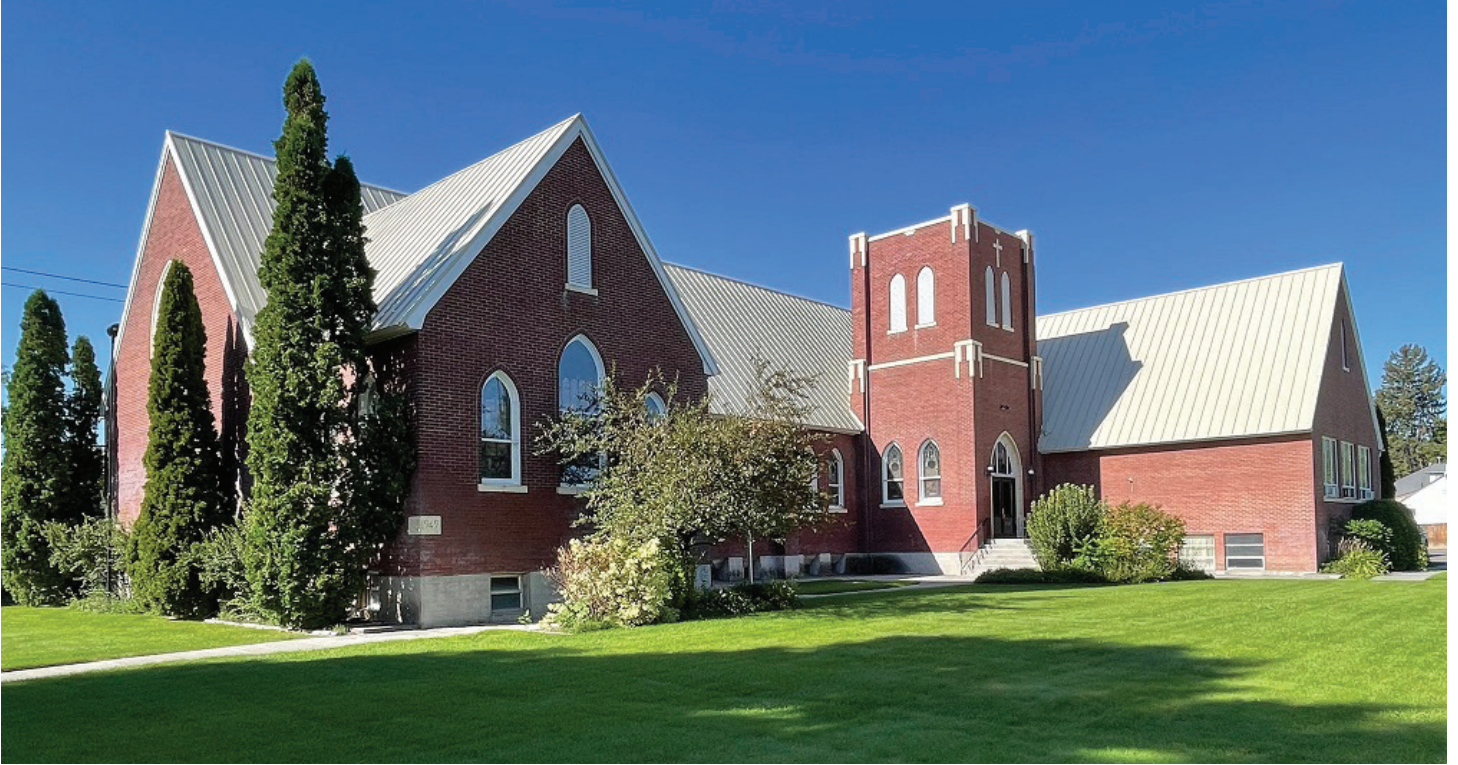
St. John Lutheran Church Idaho Falls, ID (NRHP #100009872)
